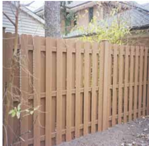
8. Wood privacy Board-on-Board
